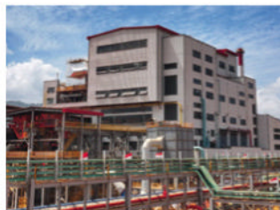
RKEF Line I Smelter. Photo: Ceria Corp
